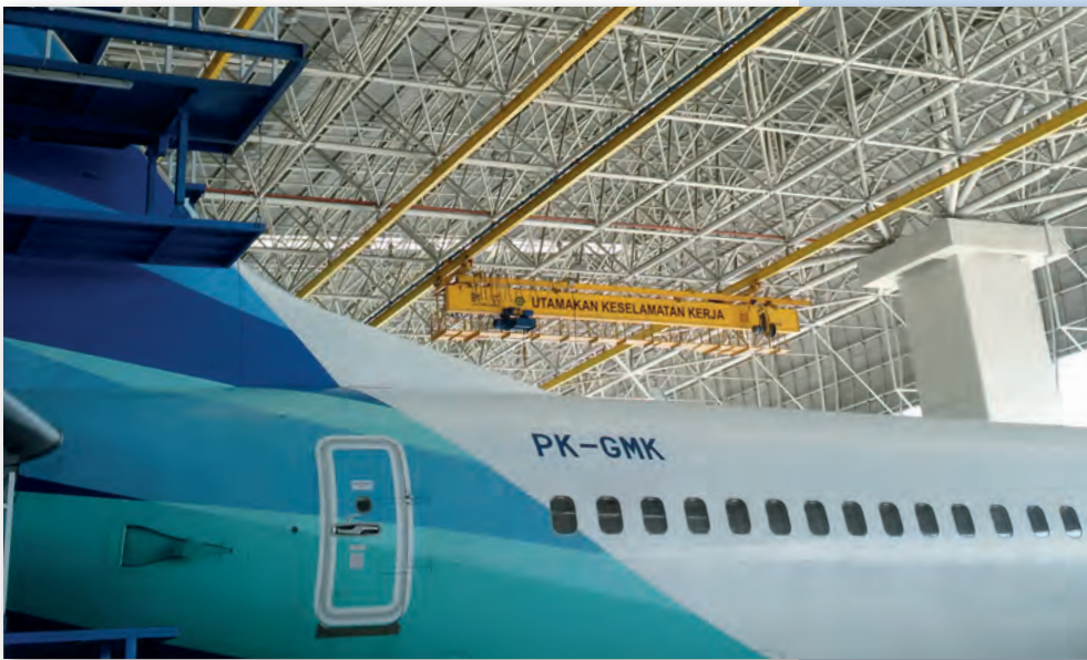
Hangar aeroportuali Airport hangars
